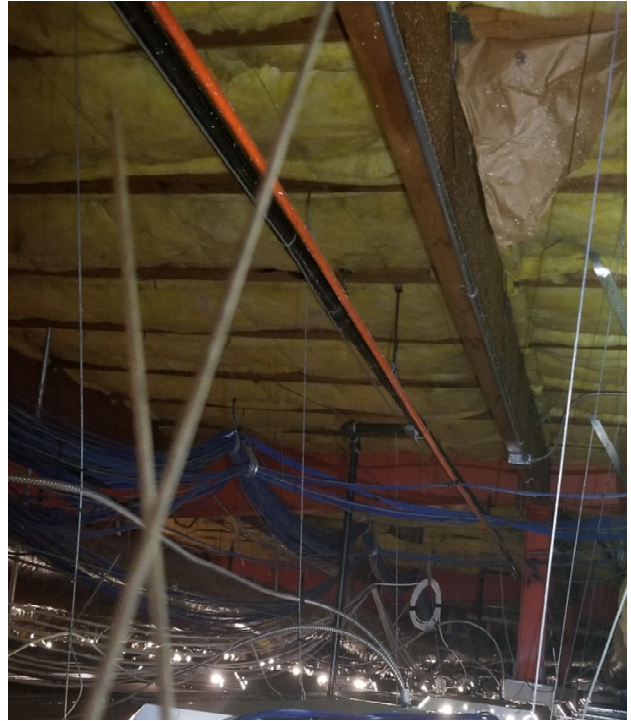
Figures 1&2: Roof/Floor framing: steel post and girder with wood beam
