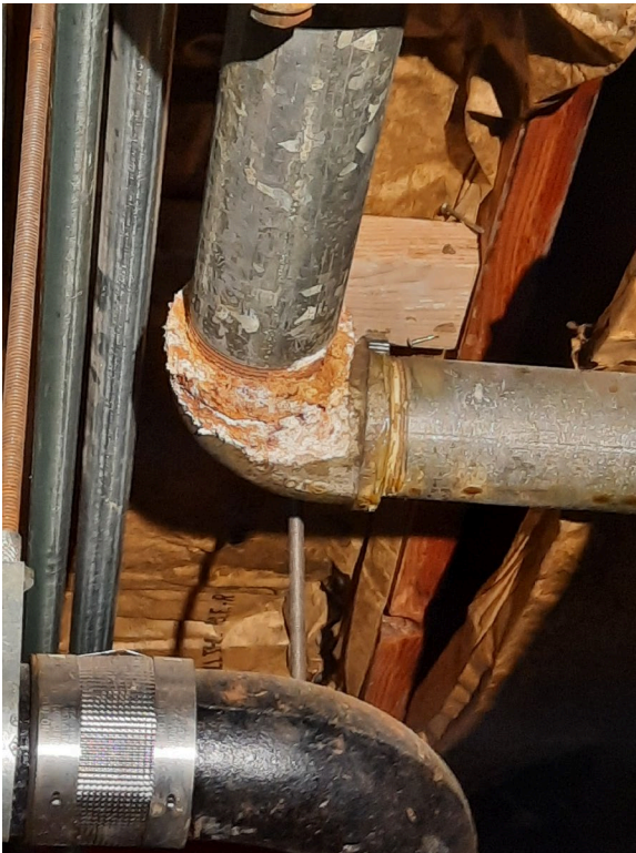
Photo #20 Old galvanized pipe showing corrosion.
