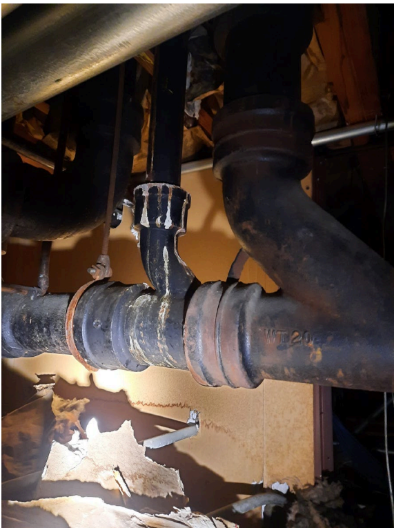
Photo #18 Cast iron pipe with some corrosion at joint.
