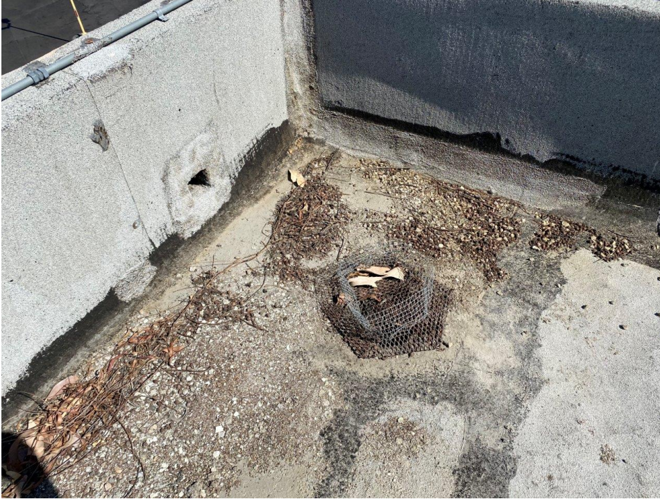
Photo #7 Roof Drain – Note the overflow and screen.
