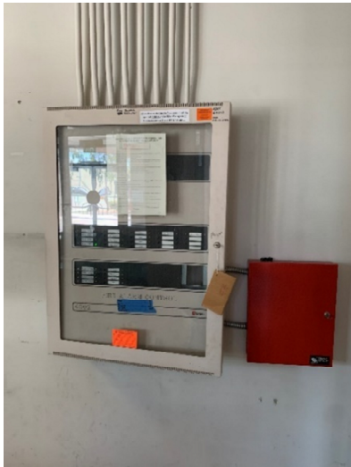
Existing Main Fire Alarm Panel
