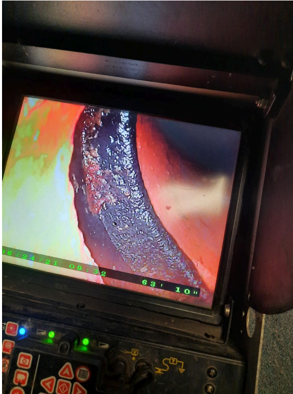
Photo #13 Clay pipe interior. Note separation at joint.
