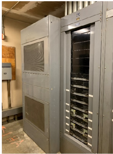
Transformer attached to Switchgear
