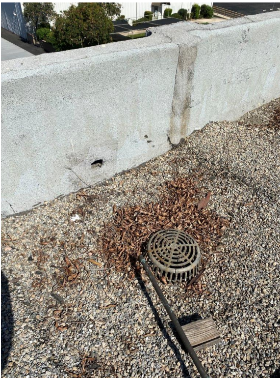
Photo #8 Roof Drain – Note the overflow.
