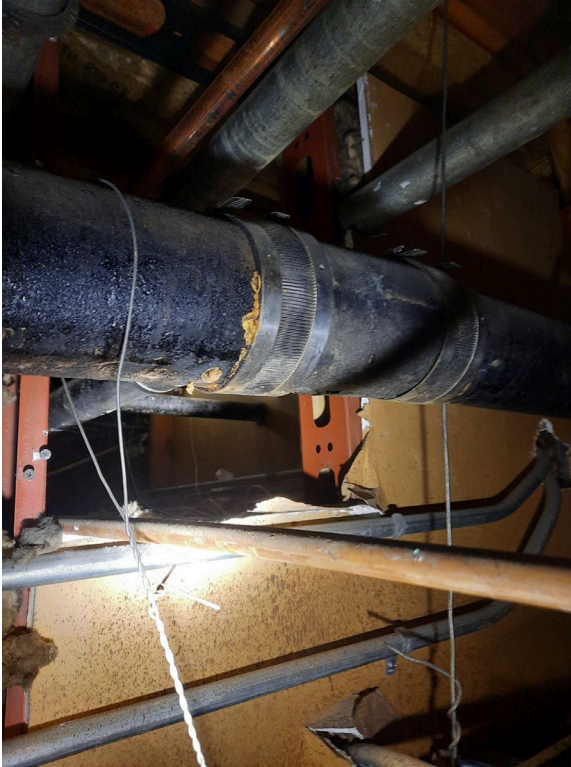
Photo #17 Cast iron pipe with minor corrosion at joint.
