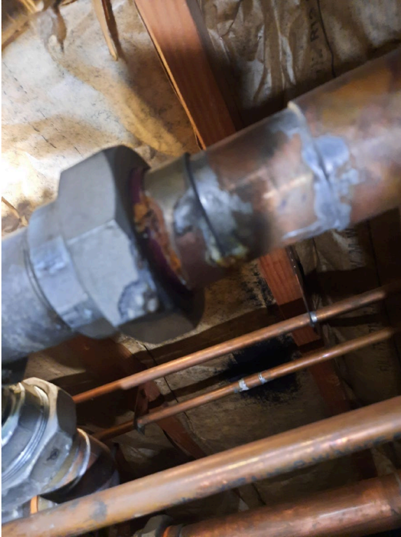
Photo #19 Old repair joint between original galvanized pipe and newer copper pipe
