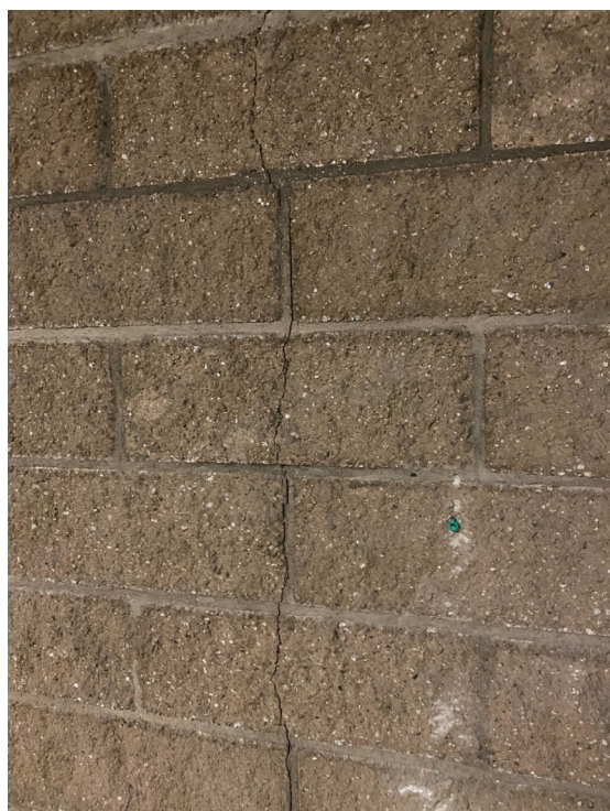
Figures 9&10: Cracks on the masonry and concrete wall
