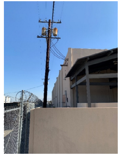
Utility Transformers on Pole
