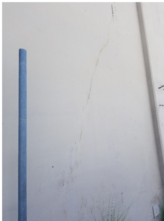
Figures 9&10: Cracks on the masonry and concrete wall
