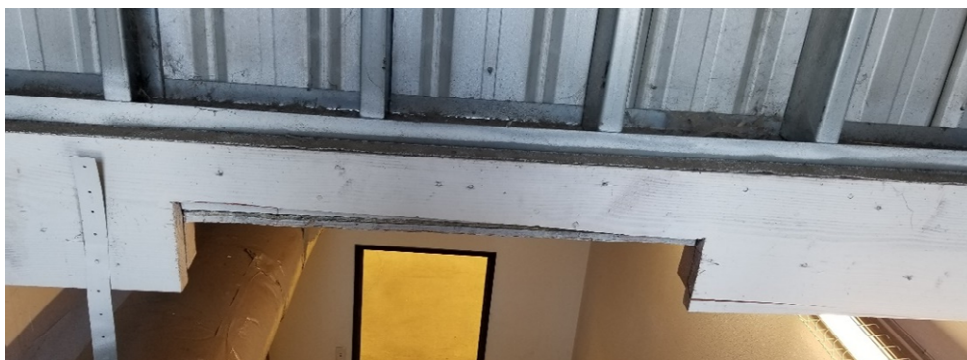
Figure 7: Cut out beam section
